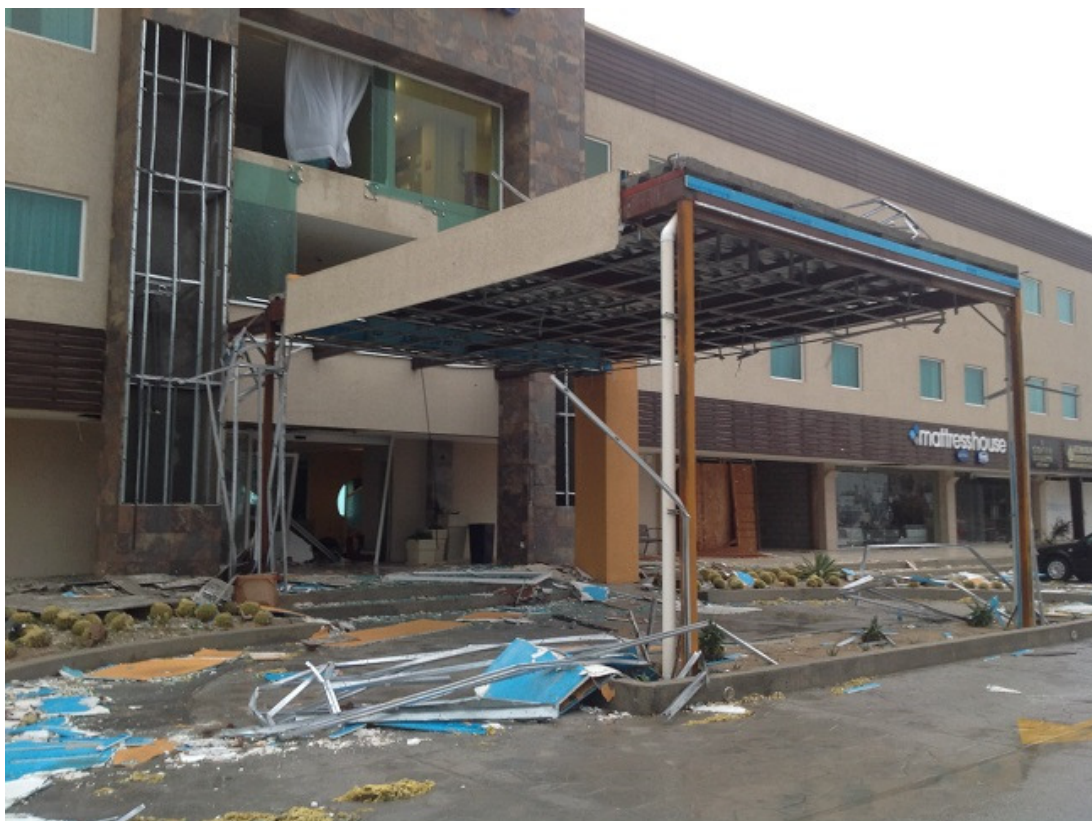
Exterior front entrance of our hotel the next morning. The hotel faces N, and most of the damage to the front of the building—smashed windows, destroyed entrance, collapsed facades, and shredded pillars and portico—happened during the cyclone’s front side.
