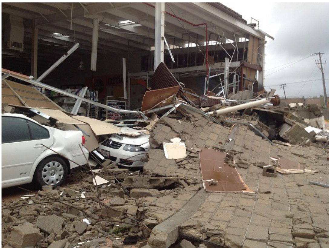
The Office Max next door to our hotel partially collapsed, burying nearby cars. The walls were made of cement blocks, with steel rods running through them.
