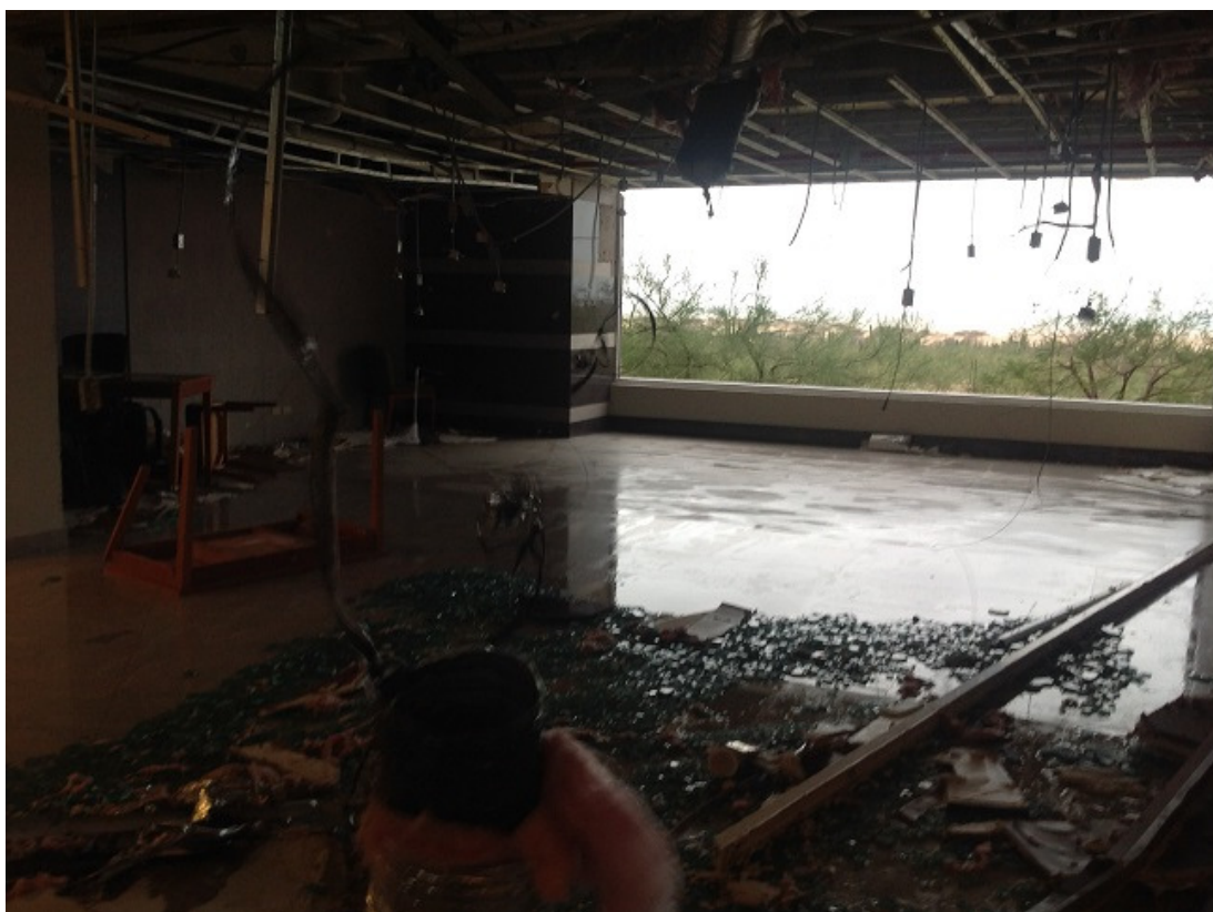
The rear glass wall of the lobby (facing S) completely blew out as the cyclone's backside swept in after the eye, turning the lobby into a wind tunnel. Powerful winds then gutted the interior.
